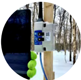
Monitoring system installation
